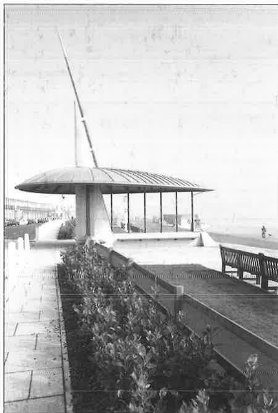
Dover seafront improvements
