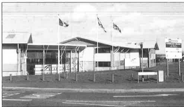
Business development on Phase I, White Cliffs Business Park
