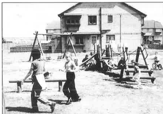
Children's play space provided as part of new development
