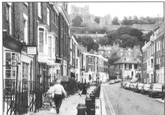
Castle Street, Dover - a popular location for offices
