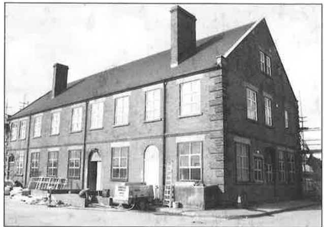
Former colliery offices, Betteshanger Colliery
