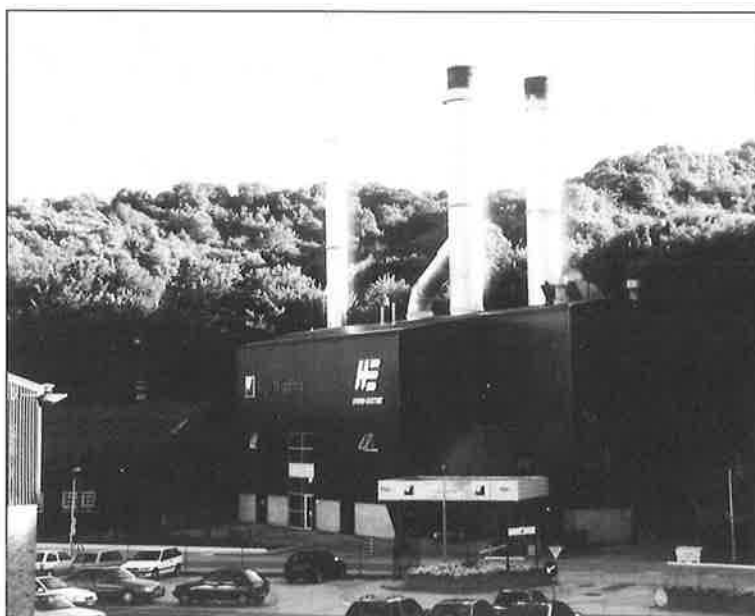
Combined heat and power plant, Dover
